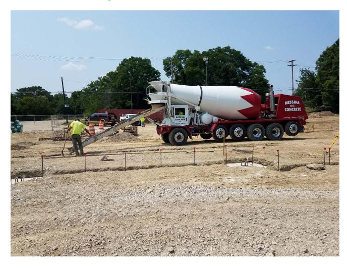
Concrete placement for building addition foundations.
