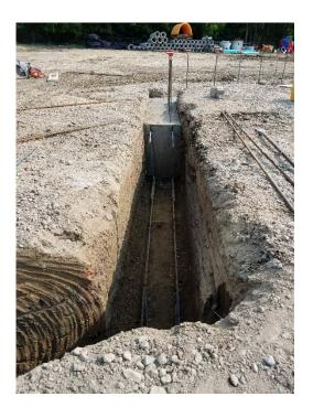
Installation of foundation reinforcement bars and placement within footings.
