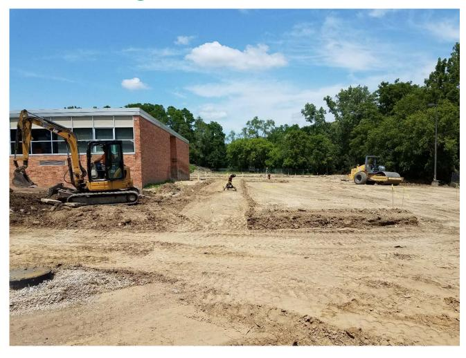
Parking lot & sidewalk subbase, prior to stone and asphalt placement.
